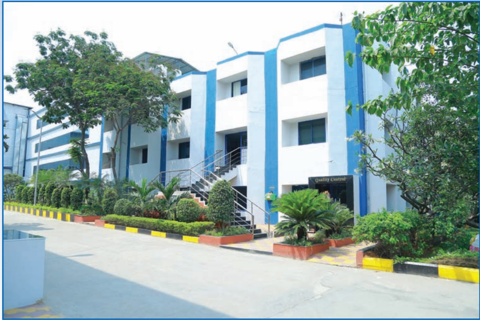
New Quality Block in Unit 1, Kazipally
